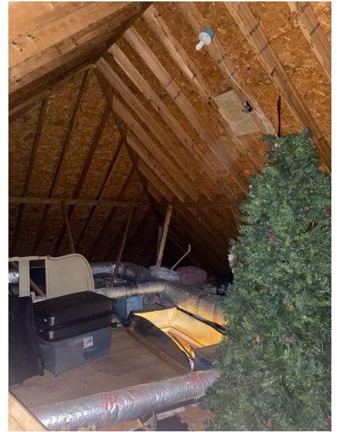
Attic Access: Access Type(s) Pull Down Stair(s)
