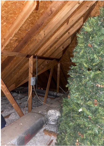
Inspection Method: Amount of Attic Visually Accessible 80-90%
