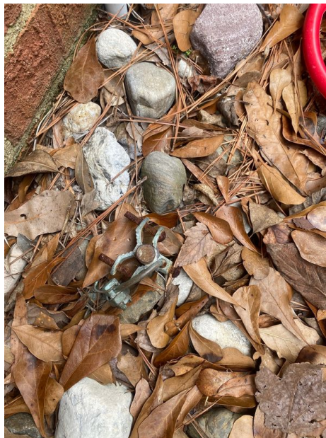
Branch Wiring : Visible Branch Wiring Type NM Sheathed Cable
